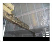
the role of tight barrier plasterboard ceiling. It must be scrupulously rigorous on its application and on the junction of these positions. Ask waterproof electrical boxes. The shear walls are also great sources of leaks and thus treated by the projection of a aéroblue. To the junction with exposed beams, again you have to be very careful about applying a seal between the support rail and the beam and rail and also place. Attention to all sanitary and electrical penetrations.
