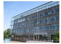
according to the terms of environmental regulatory, bioclimatic skin turns cold climate near the surrounding when it's hot and warm when it's cold. And the buffer space created between the glass skin and the existing façade allows energy performance and occupant comfort. In addition to maintaining the large openings of the buildings without reducing their surfaces, we make generous natural light in all classrooms while renewing the interior comfort without changing the medium.
