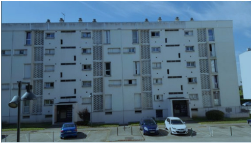
The residence before work - photo credit: TerreEco
