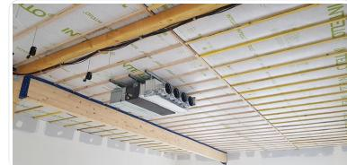
Ease of adaptation for the installation or modification of non-partitioned offices with regulation by rooms or areas. The use of flexible sheaths makes it easy to change the location of mouths in case of new partitions unlike commonly used systems.
