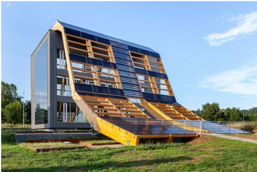
The photovoltaic pergola on the main south facade marks the entrance to the building, with a dual function of solar filtration and energy collection.
