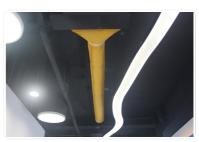
A kind of flexible air distribution system woven from special fibers, the fabric air supply system is mainly used to replace traditional air supply pipes, air valves, diffusers and other air supply systems, and has been widely and
