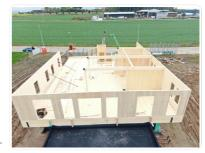
Posts-Beams mixed structure STABILAME in glued laminated
