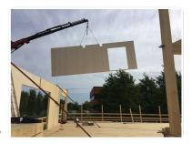
Mixed post-beam-CLT structure
