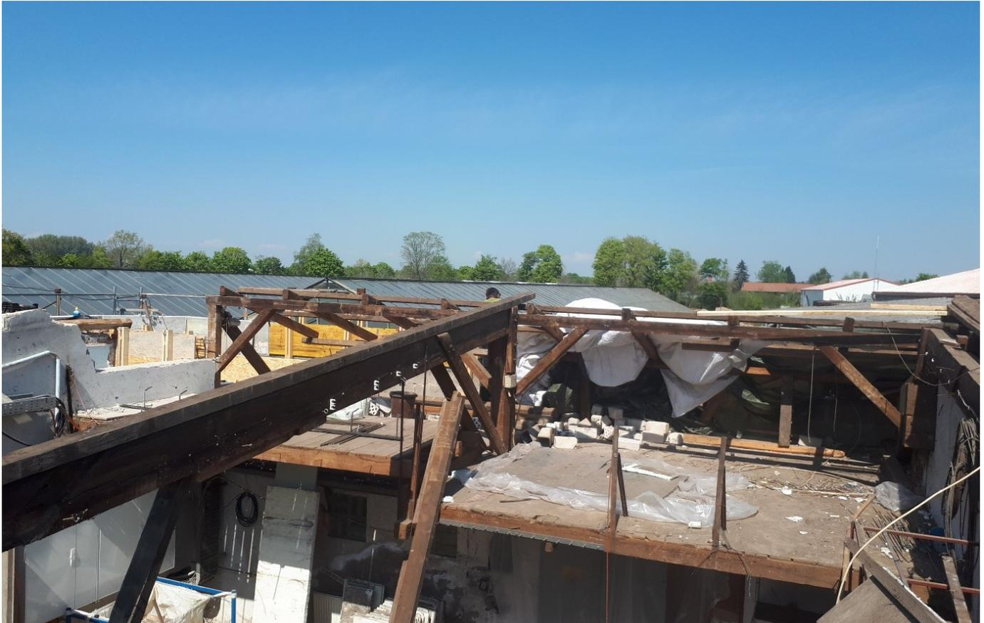
Figure 6 Underlying roof structure after the removal of the corrugated roof plates, visible is the crawl space which will later serve as the technic room for the rooftop greenhouse
