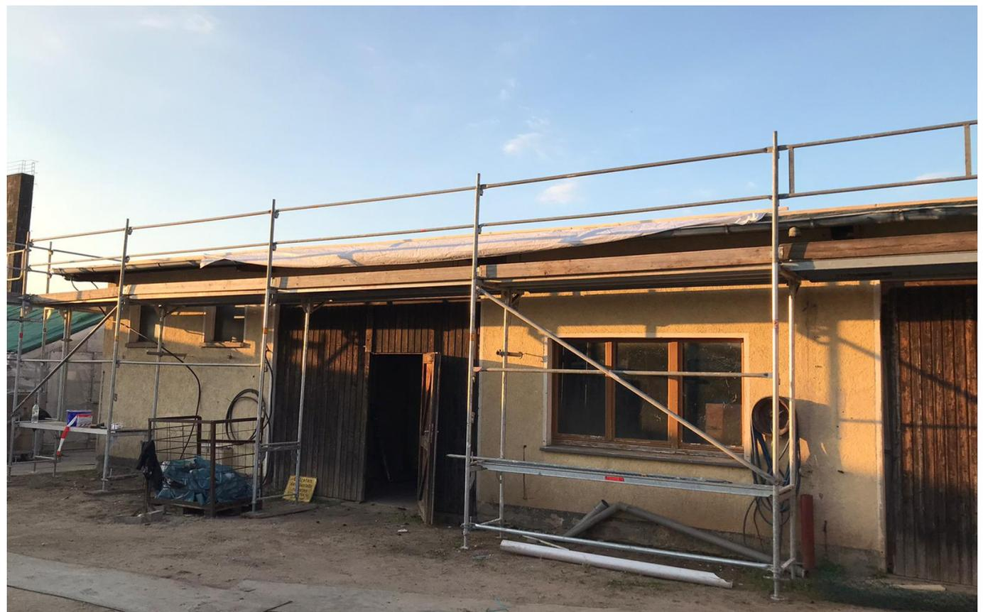
Figure 5 Support building surrounded by scyffolding, roof covering already removed
