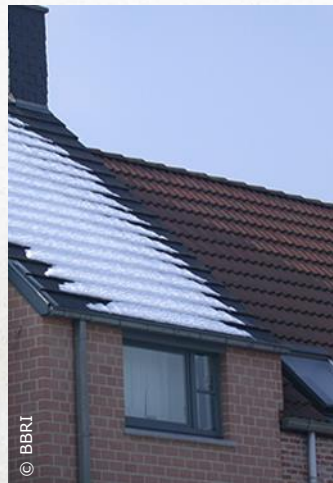
Insufficient insulation
