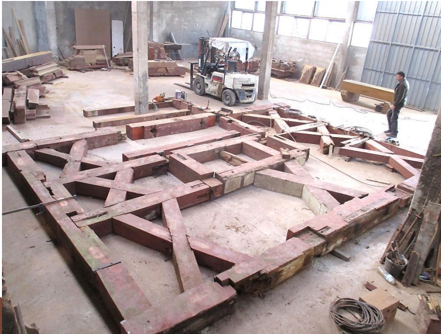
Rehabilitation of the bell heads and bell support structures
