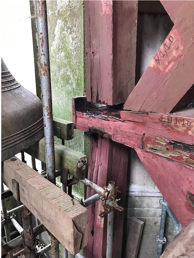
Degradation of the bells timber support structures
