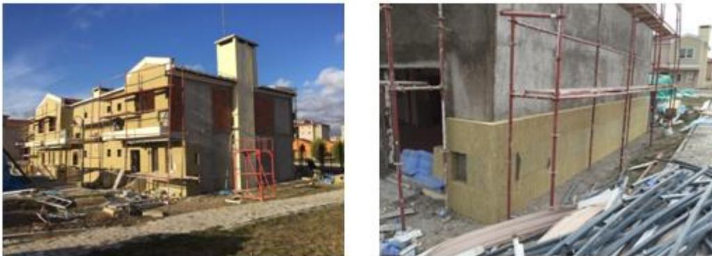
Figure 1 External insulation implementation in Tepebaşı demo site
