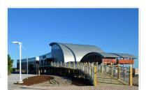
The building is also equipped with zinc shingles and thick, galvanized-coated steel resistant to corrosion from salt spray.
