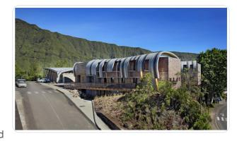
or concrete; • a FOAMGLAS® cellular glass insulation panels (T4, S3 or TAPERED) grouted with bitumen and glued to the support; • an attachment interface having galvanized steel plates engraved to FOAMGLAS® and a SBS modified bitumen membrane welded to the FOAMGLAS® and covering the pads; • a cover zinc standing seam (width of single out 430 mm) made using VM ZINC PLUS sheets (polyamide with polyurethane coating 60 J.lm the
