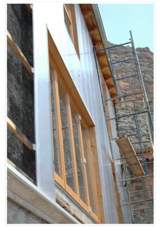
reflection on the polycarbonate there is virtually no refracted solar radiation or visible radiation entering the wall in summer: the wall is not heated when the sun is high or summer. On the
