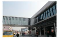
Outdoor shading aluminum board is mainly located on the outside curtain wall of the corridor lounge of terminal
