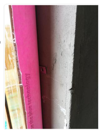
heat-breaking bridge anchor
